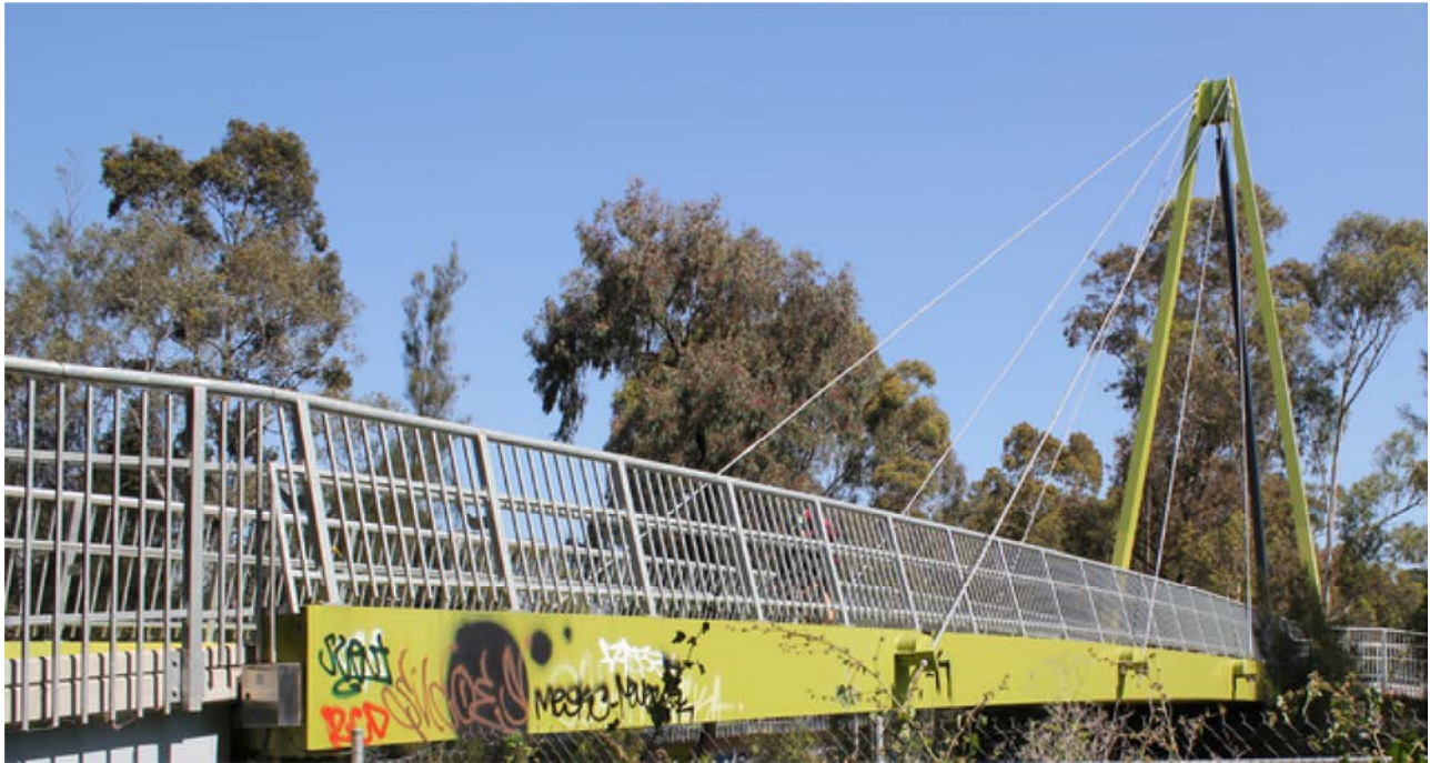
FIG. 1: Pedestrian bridge used as a model for the design project
