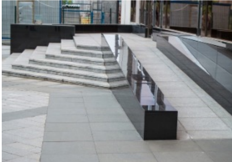
FIG. 1: Building entrance with stairs and a ramp for people who use a wheelchair at a large modern office building, store. Getty images copied under license.
